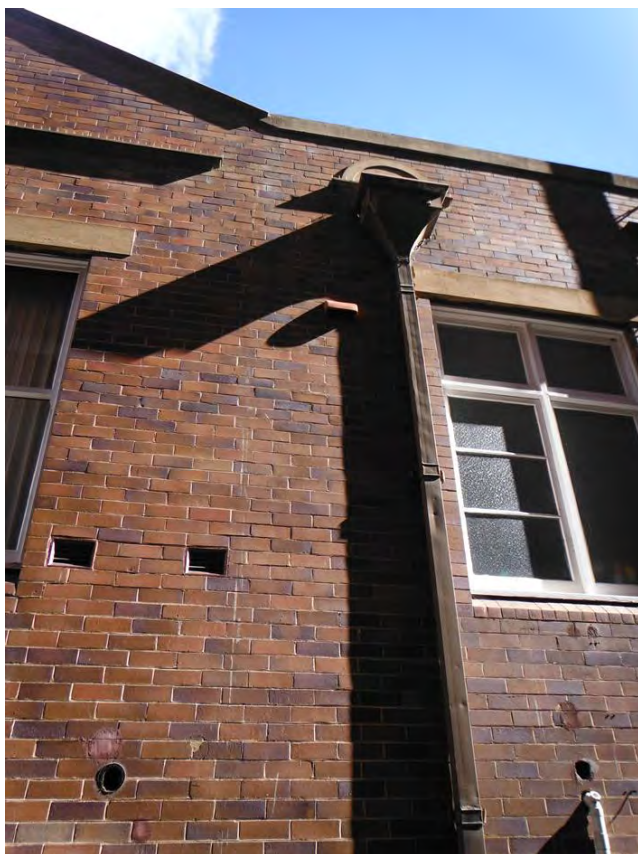
Fig. 123 Detail of box gutter and decorative stone work above gutter , north side of Town Hall [Author's own photo, 7 September 2017]
