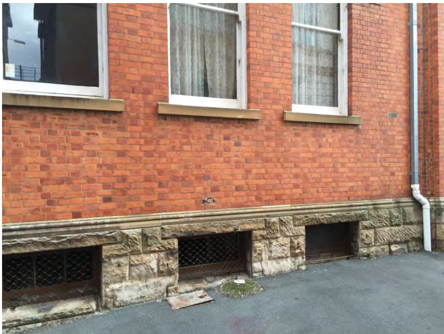
Fig. 87 Detail of stone footings, air vents and foundation at base of Town Hall (1887)
