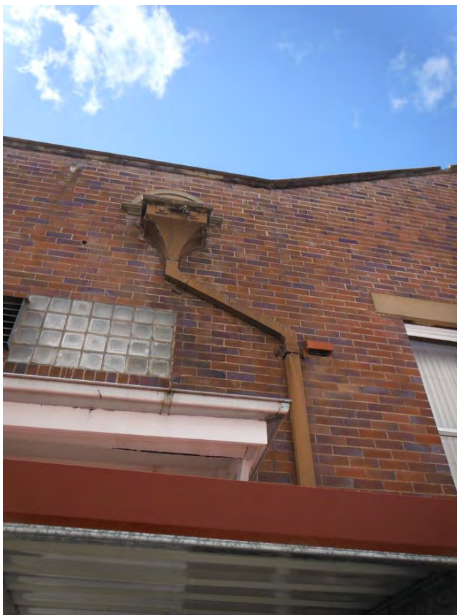
Fig. 122 Detail of box gutter and glass brick window, south side of Town Hall
