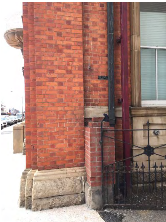
Fig. 85 Detail of corner of Town Hall facade showing brickwork, sandstone foundation and decorative Iron Gate (south side)
