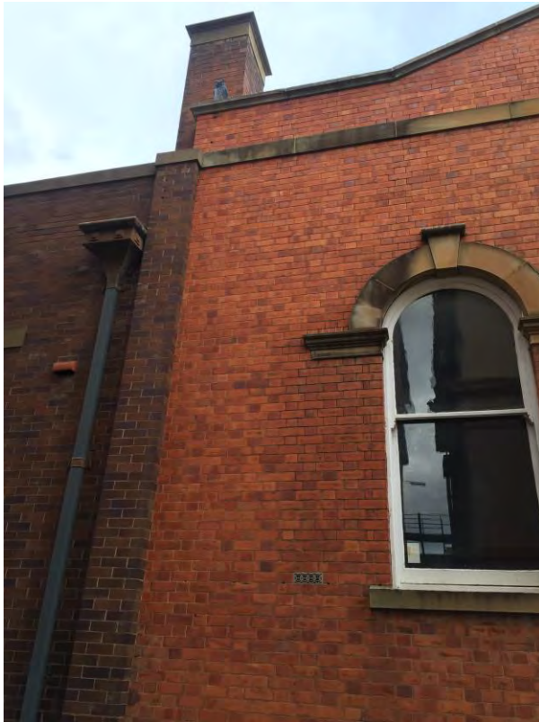
Fig. 86 Detail of south side of the building; detail of box gutter, window, 1887 brickwork and 1936 brickwork join
